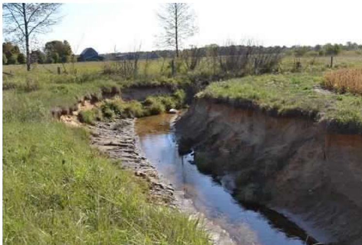
Figure 6. Bank erosion involves the undercutting and scouring of natural stream and drainage channel banks.
